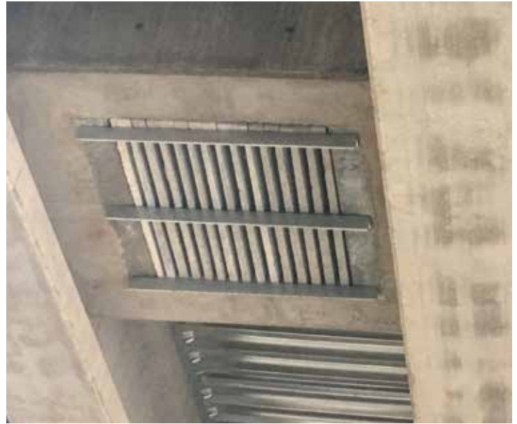
New bat boxes under the Ina bridge, Arizona Game and Fish Department
