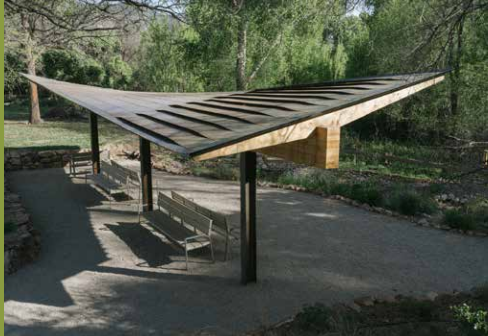
Viewing Pavilion completed 2018, Logan Havens
