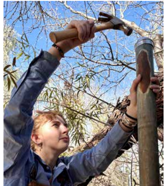
Nicole Marking shows how easy it is to tap inexpensive metal caps on open fence posts, eliminating their danger to wildlife.
