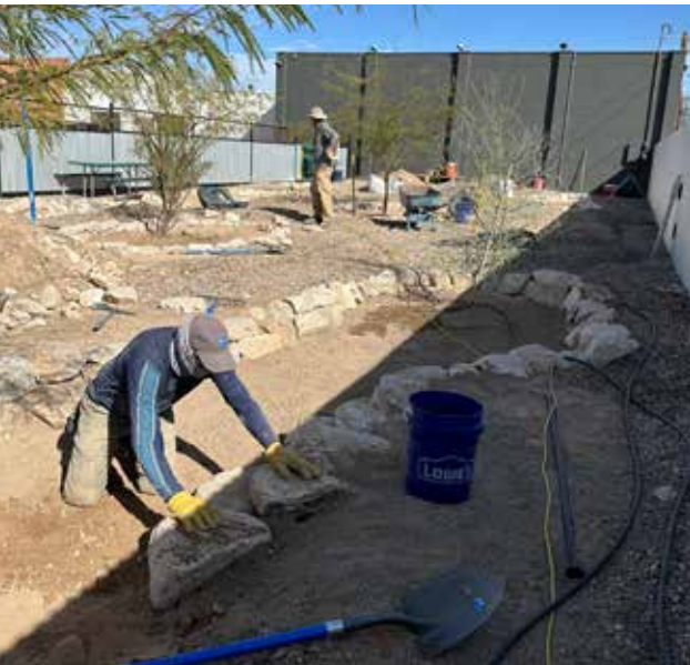
Field crew member Dan Lehman lays rock around a rainwater basin. This helps to prevent erosion.
