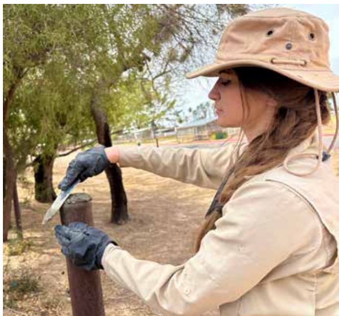
Olya Weekley, Applied Conservation Program Manager, uses cement to seal an older fence post with an opening too large for a standard-size metal cap.
